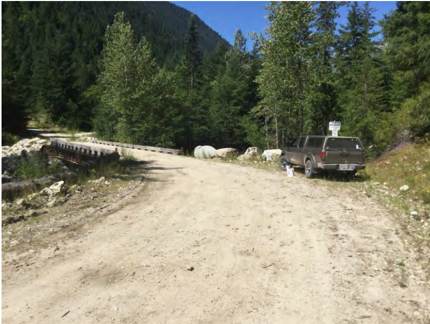
Left Approach Facing Bridge
