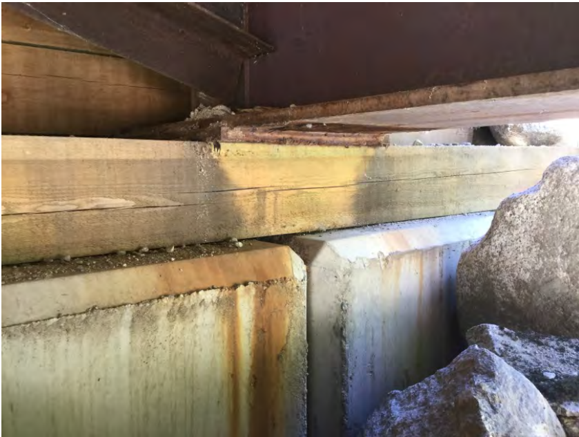
Typical Girder Bearing on Sill
