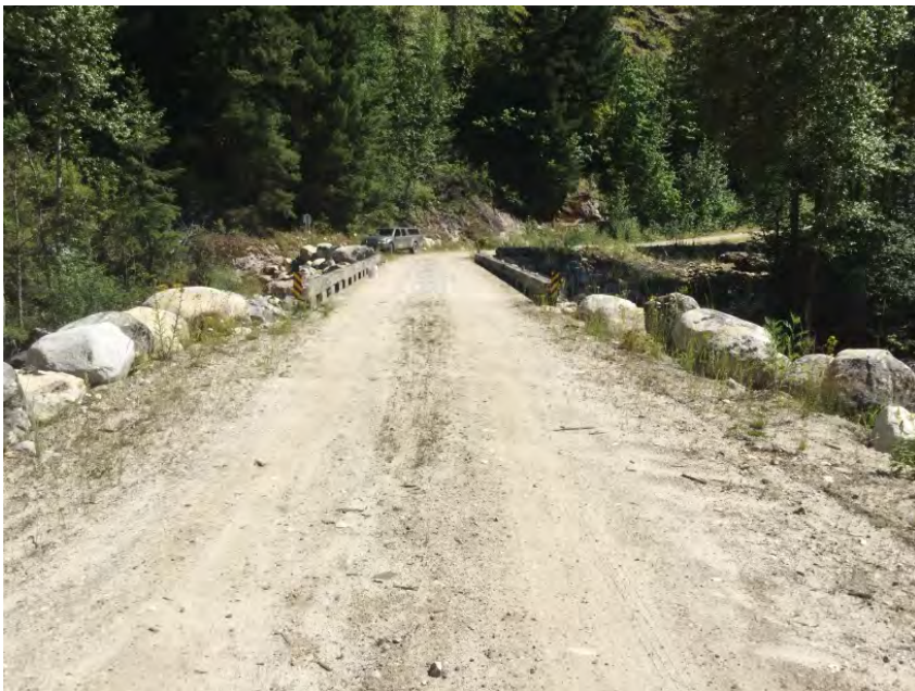
Right Approach Facing Bridge
