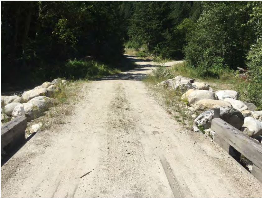
Right Approach Facing Away From Bridge
