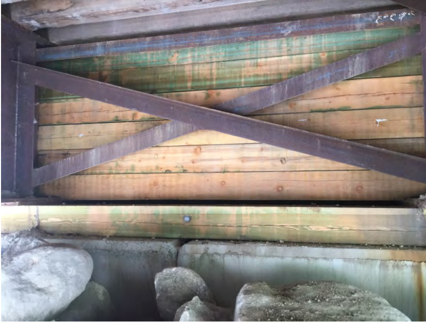
Typical New Sill & Lock Blocks
