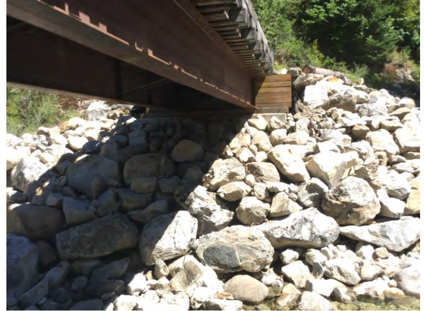
Left Bank Abutment
