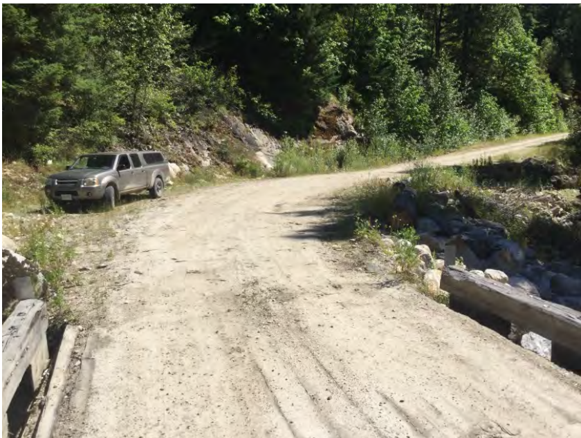
Left Approach Facing Away From Bridge
