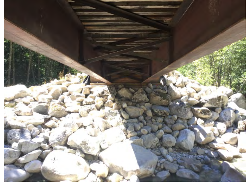
Right Bank Abutment
